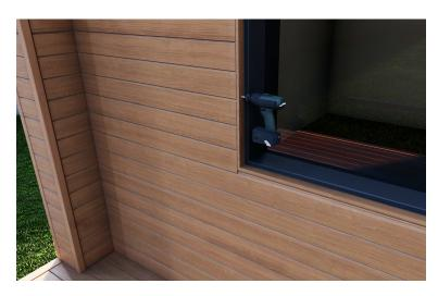
11. Fascia Boards can also be used for finishing around window and door revels. Cut the fascia boards to size and pre-drill holes before securing. Slowly tighten to prevent cracking of Boards. Colour coded screws can be used for this application
