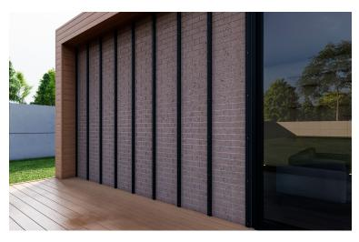
3. All battens need to be flat and level against the wall. Make sure you use a spirit level to check levels before fitting the boards.
