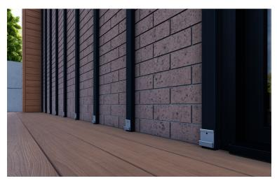
5. Attach a Starter clip to the bottom of each Batten, this will give the first Cladding Board something to clip into. Ensure that each clip is level with the next and that the first Board sits level on the clips before continuing to the next step. It maybe necessary to give the top edge of the cladding board a tap to ensure its fully seated in the starter clip.
